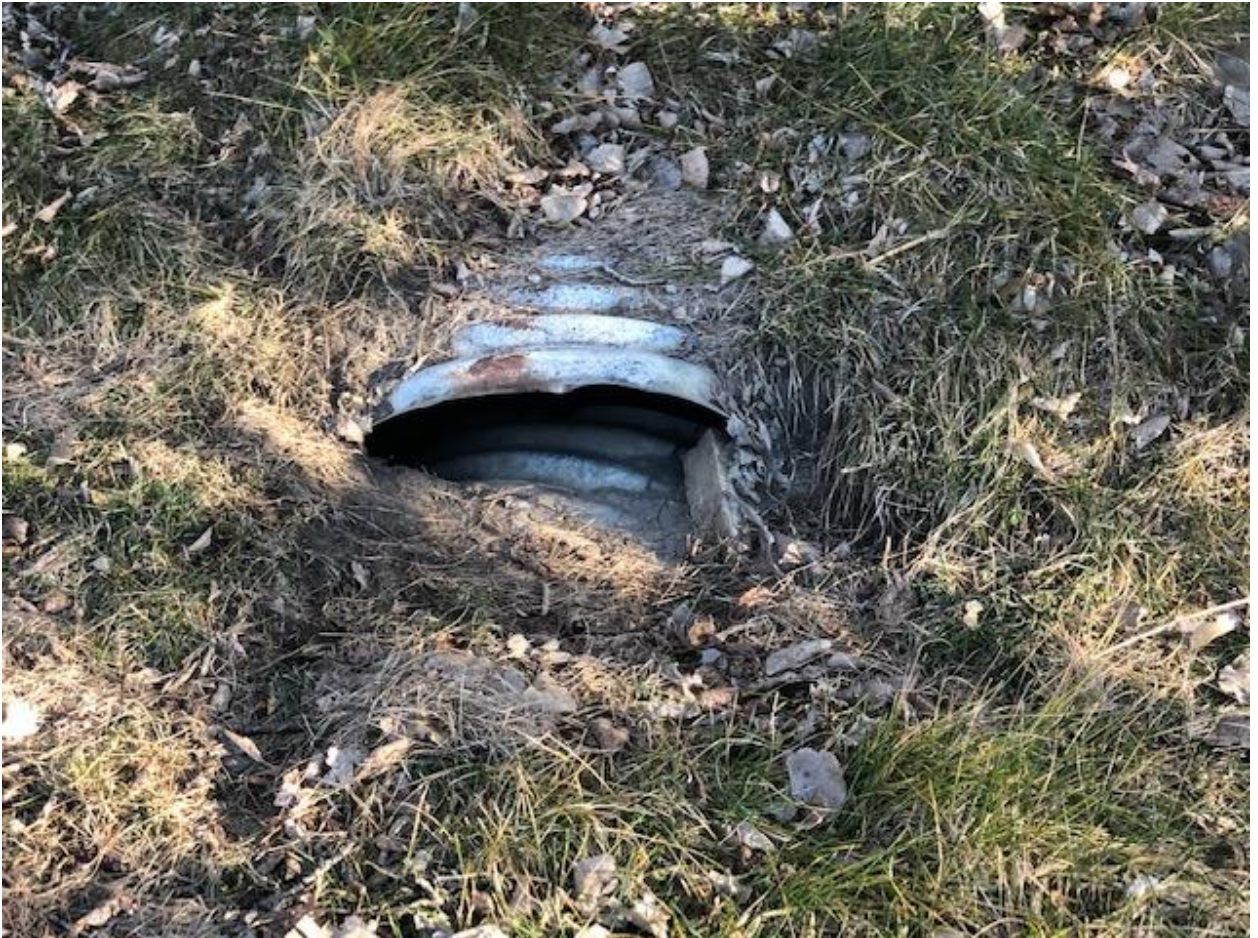
Existing Weber-Stephens side of railroad culvert.
