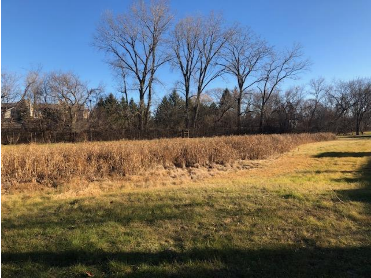
Existing storm detention area. Very overgrown causing water conveyance issues.
