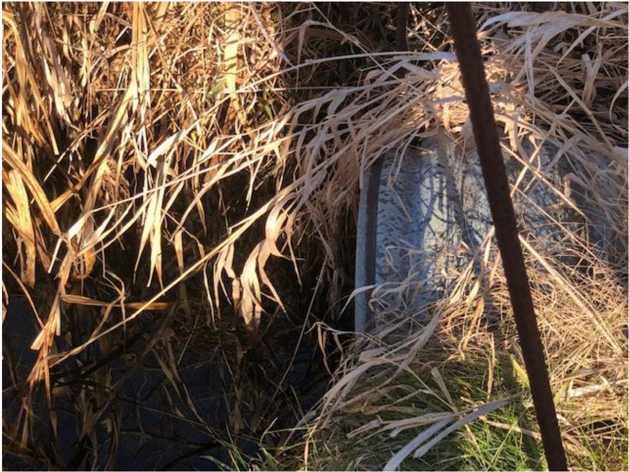
Existing storm pipe inlet into detention area.
