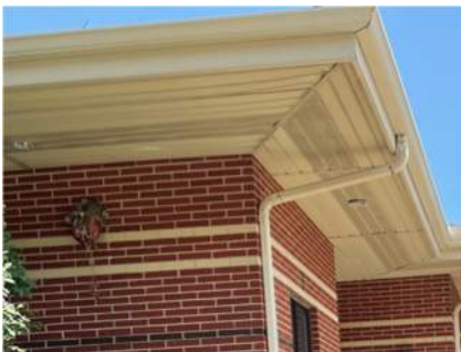
Aluminum Fascia and Soffits
