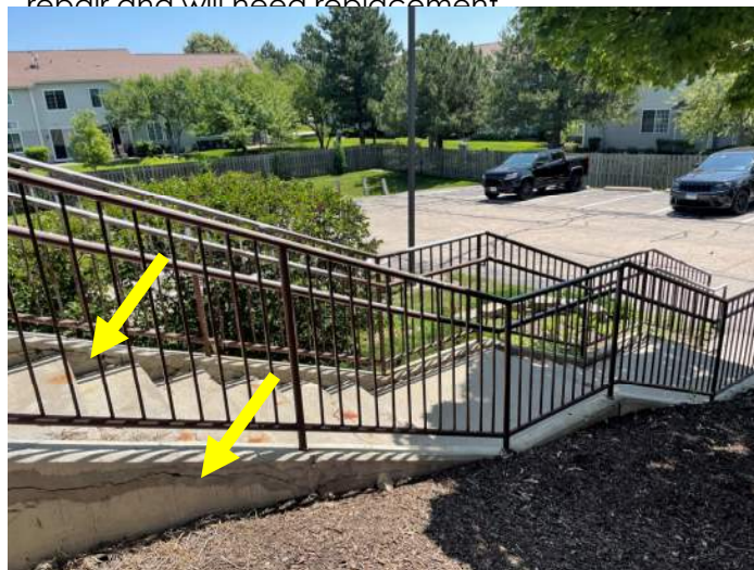
Southeast Entry Stair
