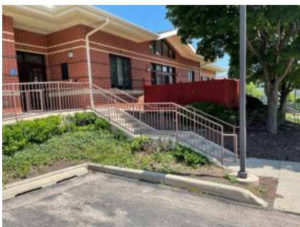
Main Entry Stair and Ramp
