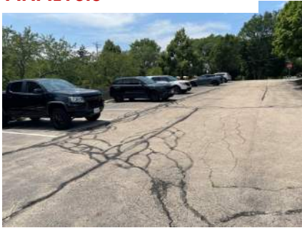
Parking Lot Pavement
