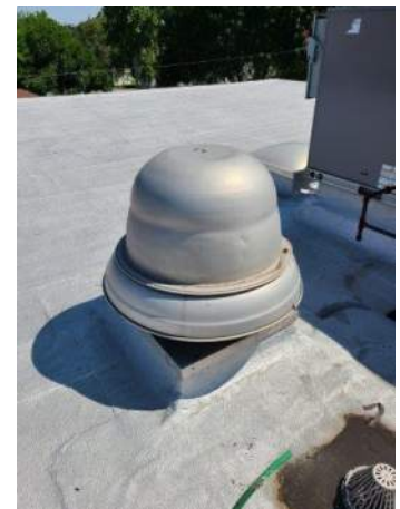
Roof Mounted Exhaust (typ.)
