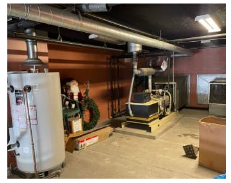
Mezzanine at Apparatus Bay
