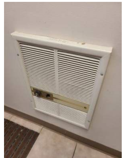
Electric Unit Heater
