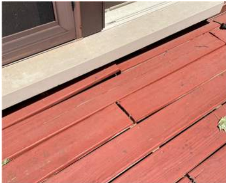
Closeup of Deck Boards
