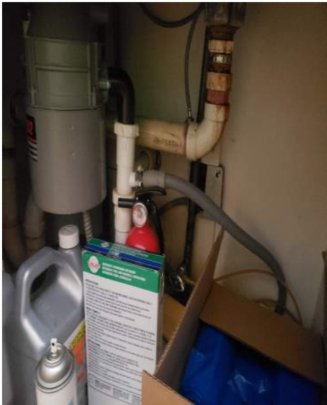
Under Kitchen Sink
