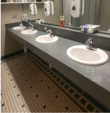
Men's Locker Room
