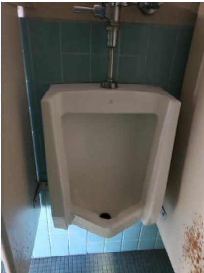
Urinal at Apparatus Bay Toilet
