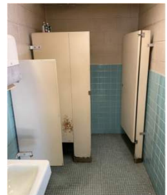
Existing Toilet Room
