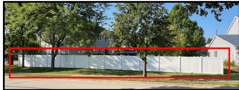
6-foot solid vinyl fence installed without a building permit, after Staff failed the building permit
