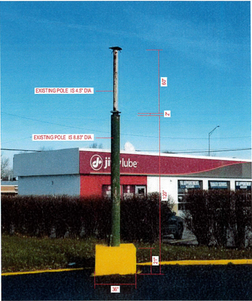
PHOTO SURVEY OF EXISTING- DUNDEE ROAD
