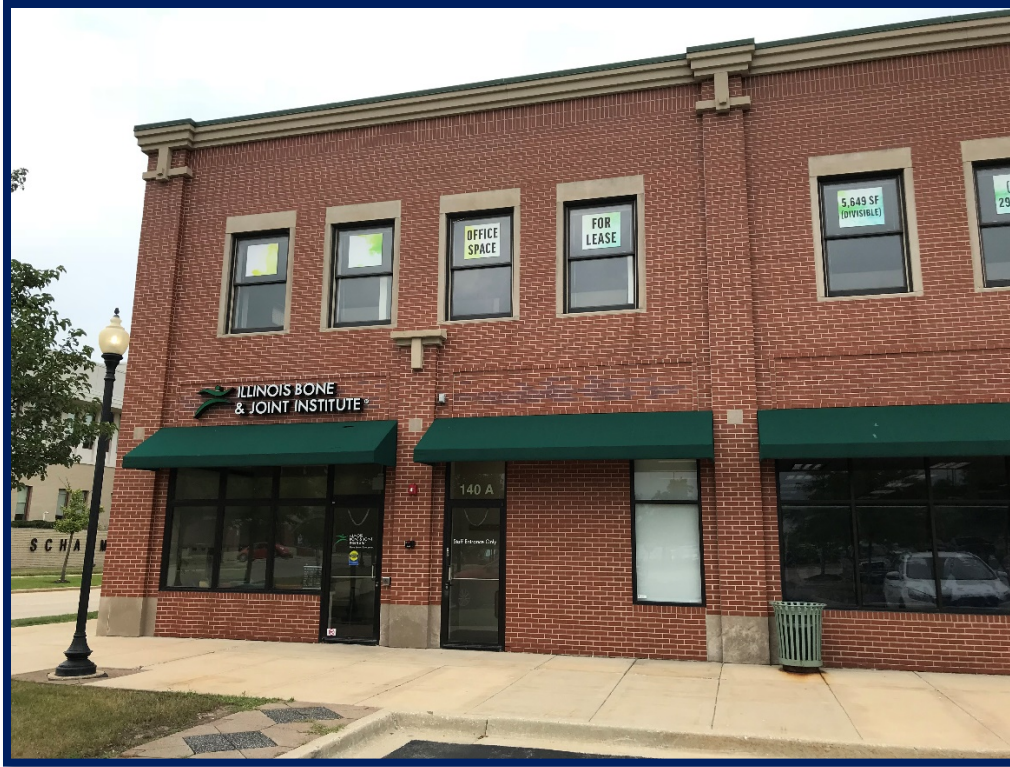
Ground View of Schaumburg IBJI Clinic
