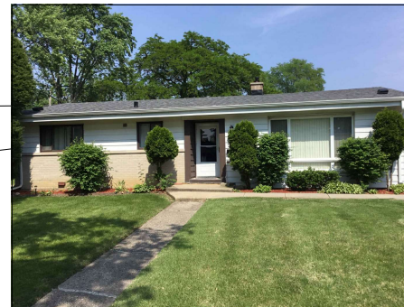
1 EXISTING RESIDENCE - PHOTO EX1.0 Scale: 1/32"
