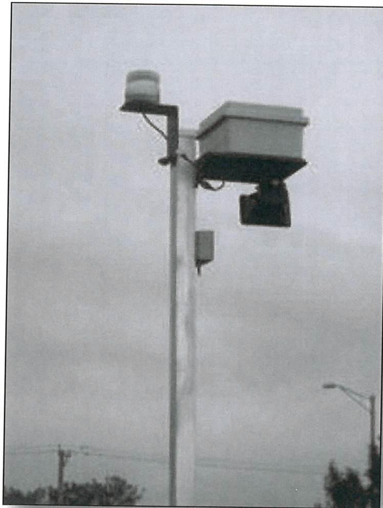
Typical "Strike Guard" Lightning Protection System
