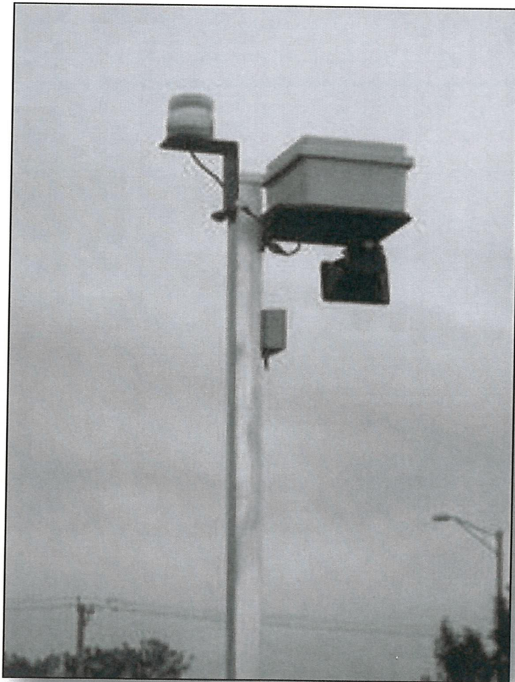
Typical "Strike Guard" Lightning Protection System
