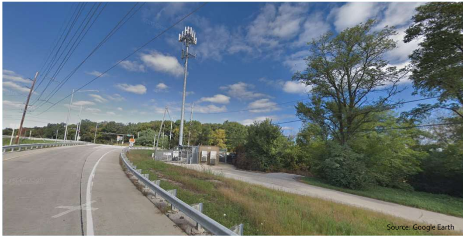
Vacant, underdeveloped parcels with a cell tower use
