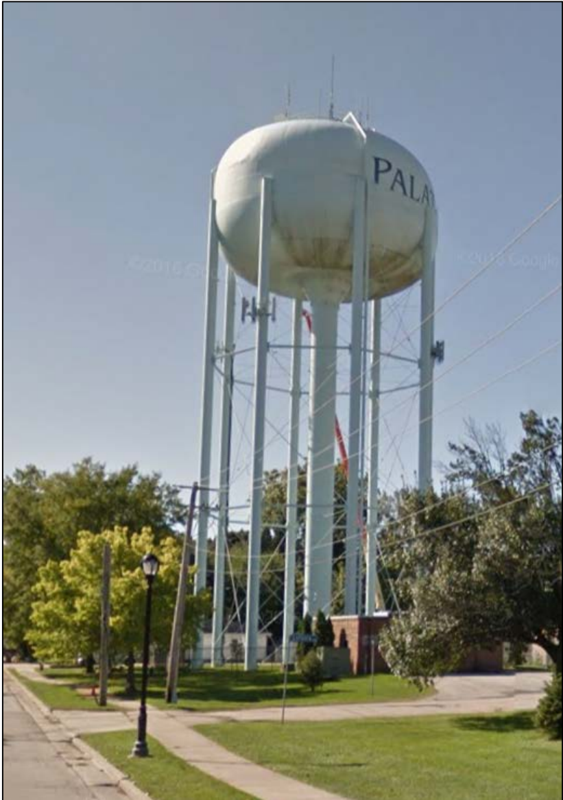
Attachment: Smith Street Tank (Smith Street Water Tower Lease Agreement)
